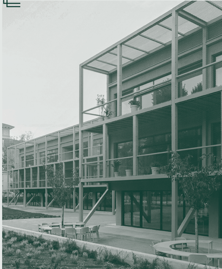
Scuola Enrico Fermi, Turin, Italy Architectural office: BDR bureau
